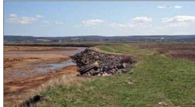
2-5 Dykes at Grand Pré are faced with rocks to help them withstand the force of tides and storms.
