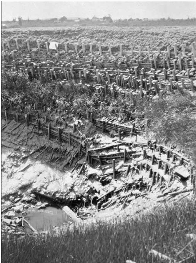
2-27 View of a 19th century aboiteau , illustrating the elaborate structure required to withstand the pressure of the tides and waves.
