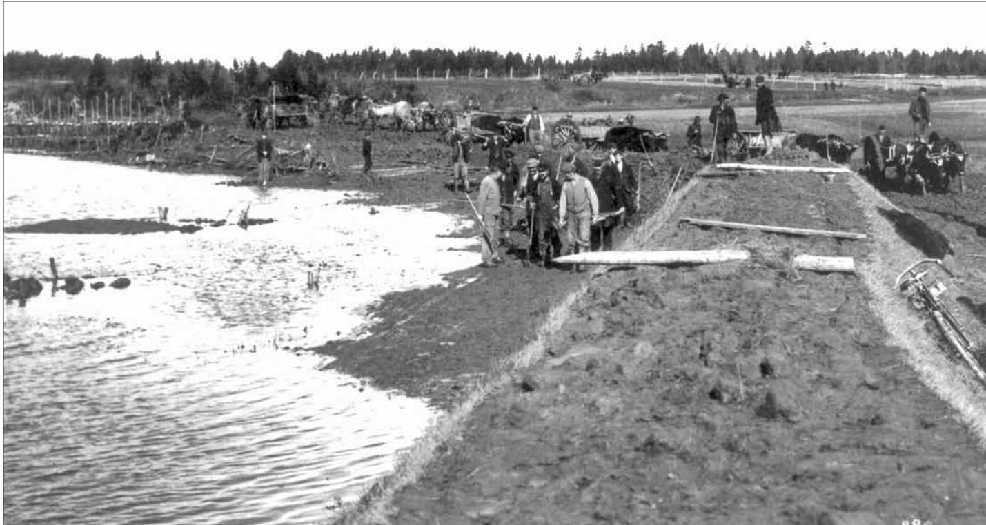
2-36 Repairing the dykes at Grand Pré, circa 1900. The tradition of building and maintaining dykelands collectively began with the Acadians and continued with the New England Planters and successive generations of farmers.
